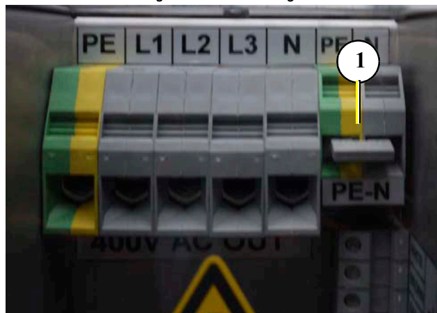
Fig. 12.9-1: PE-N bridge
