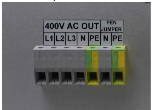
Fig. 11.5-3: PMGi AC out
