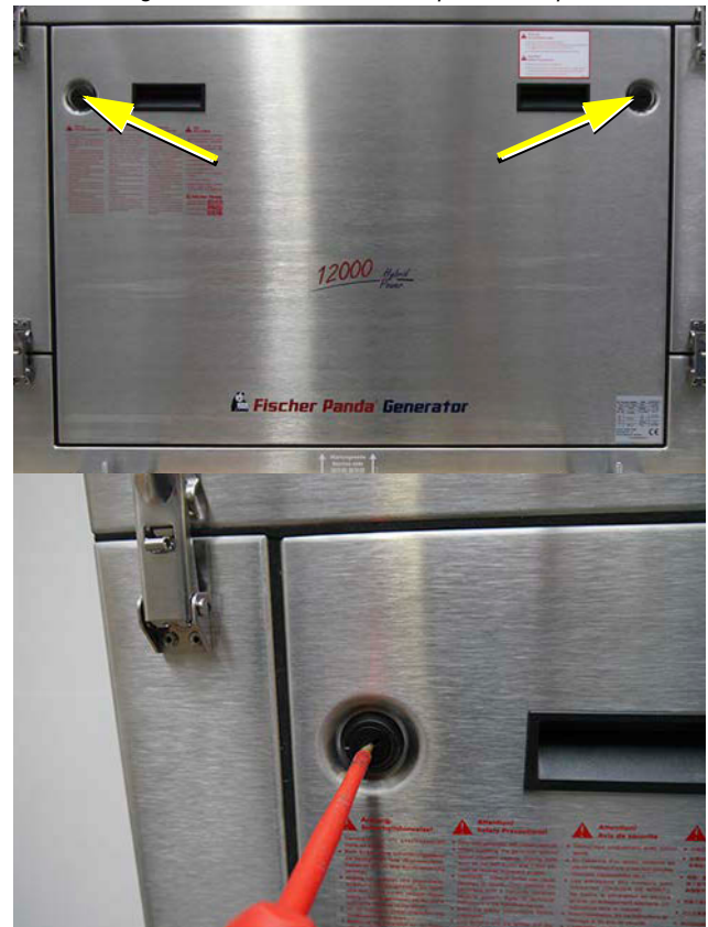
Fig. 3.5-1: Sound insulation capsule, side part
